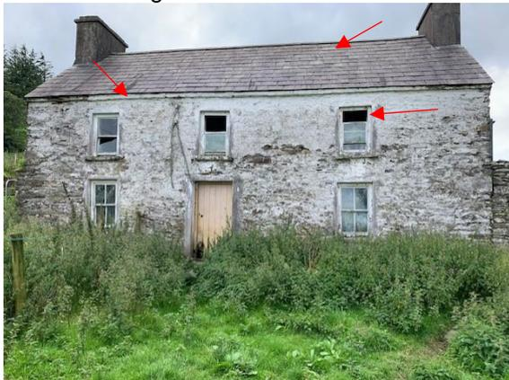
3. Derelict dwelling indicating potential access points via soffit, ridge tiles and gaps in roof tiles and open window (now demolished).
