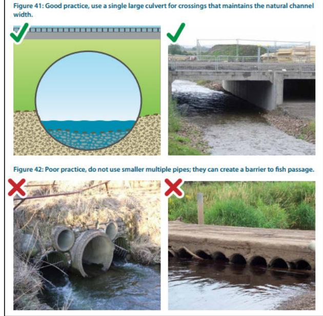
**Closed Culvert Erosion Control Good & Bad Examples – Section**
