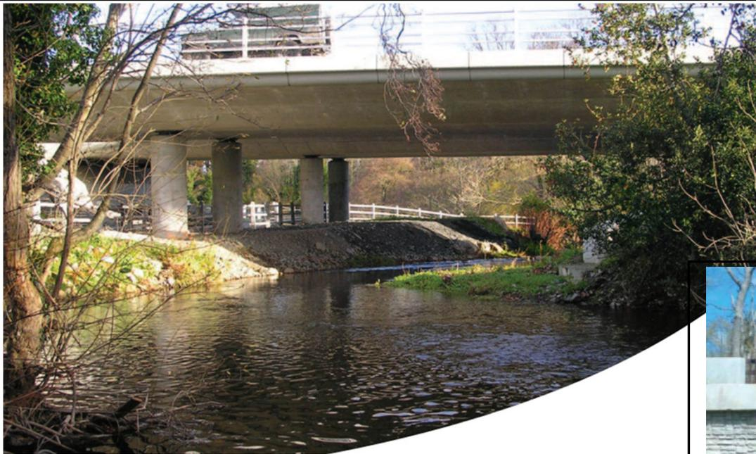
Example of a clear-span bridge which retains the existing river channel, abutments are set back from the river bank (AT&F, 2022)
