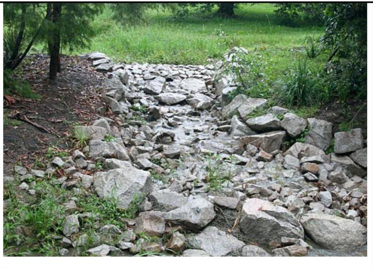
**Example of buffered outfall with coarse aggregate**
