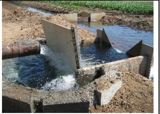
**Example of an underflow baffle in a weir pool, in practice**
