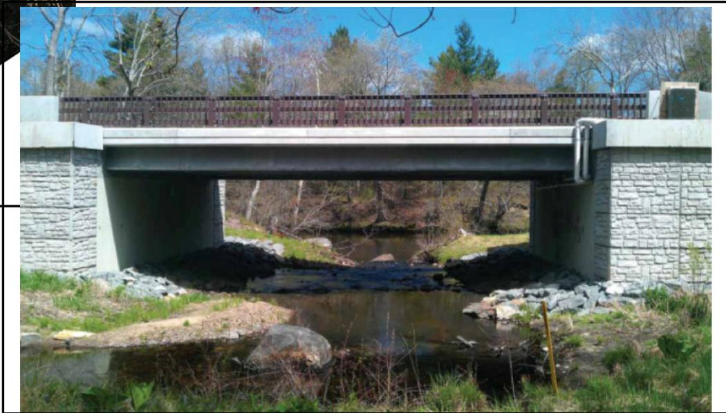
Example of a clear-span bridge, which retains the existing river channel and column set back from the river bank (National Roads Authority, 2008)
